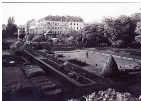
Fig. 1c. Central flower parterre and the Exhibition Glasshouse from the newly erected Karstic rockery (probably 1928): far left, below the Exhibition Glasshouse, is a smaller one (steep roof), at which place since 1985 the "Aroideae" warm glasshouse has stood. (Botanical Garden Archives)
