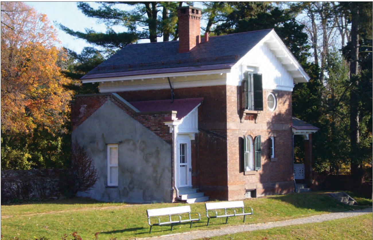
Figure 2.13. View northeast of the Gardener's cottage, an Italianate building constructed in circa 1875, which now serves as a park staff residence. The outline of the connection to the former carnation house is visible on the west wall of the building (OCLP 2008).
