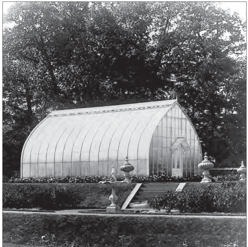
Figure 1.23. View looking southwest showing the south palm house and the statuary that ornamented the greenhouse and fountain terraces, post 1908 (enlargement of Figure 1.22). At least six late nineteenth-century Baroque style sandstone vases demarcated the walks and corners of the greenhouse terrace. Now only pieces remain. The boy and dolphin fountain was partially installed by 1906 (see Figure 1.20) and completely installed by circa 1908 (VAMA, no. V-128 detail).
