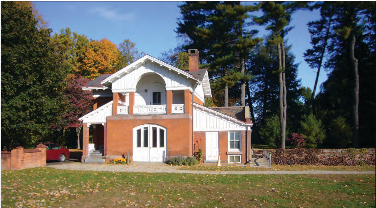
Figure 2.12. View north of the Tool House, an Italianate building constructed in circa 1875, which is now used by the FWVGA as its meeting and office space (OCLP 2008).
