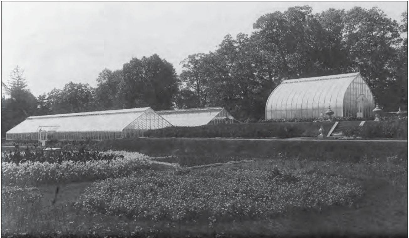
Figure 1.22. View looking southwest showing the new twin rose houses at left and one of two palm houses at right, post 1908. The fountain terrace is visible in the center of the image and the upper annual garden is in the foreground. Note the Corinthian capital in the center of the garden, which is still extant. Photograph by E. Van Osdell (VAMA, no. V-128).
