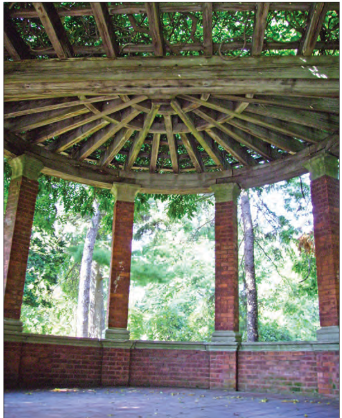
Figure 2.15. View north from within the north pergola, which is topped with heavy timbers and vines (OCLP 2008).
