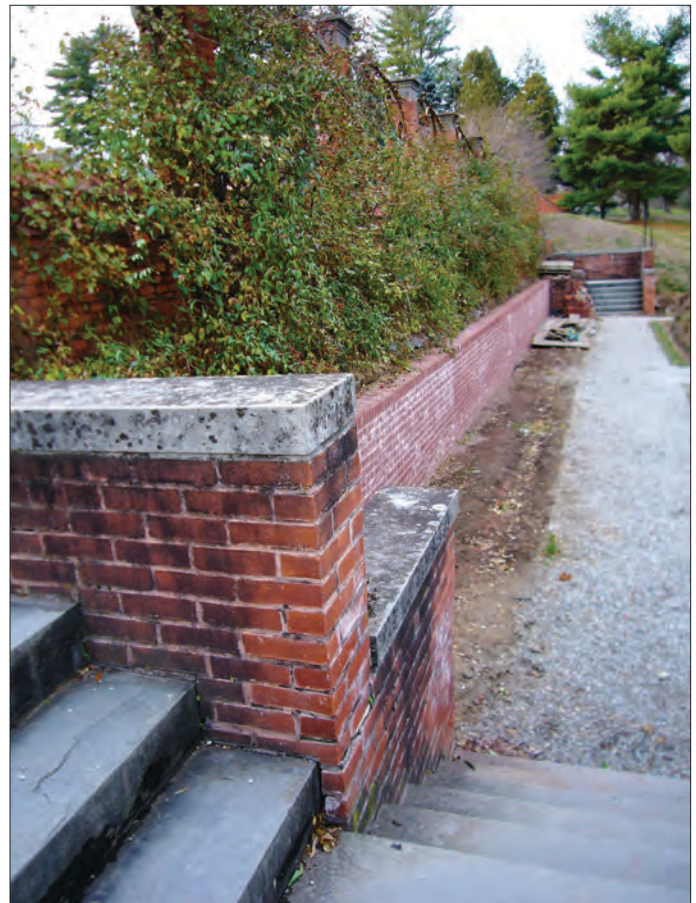
Figure 2.34. View north of the el-shaped steps leading from the lower perennial garden down to the rose garden. A recently rebuilt brick retaining wall supports a bed of climbing roses that reach the wire scrolls above (OCLP 2008).
