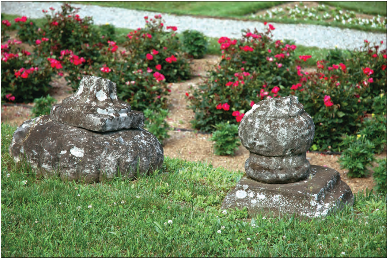
Figure 2.45. Close-up of elements of sandstone vases set along the edge of the palm house terrace. An intact vase is captured in a historic photograph on the title page. The elements are eroded and encrusted with lichen (OCLP 2008).
