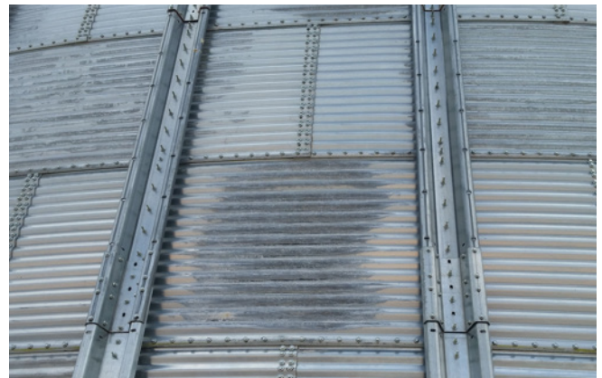
Figure 2: Example of improperly stored silo wall sheets
