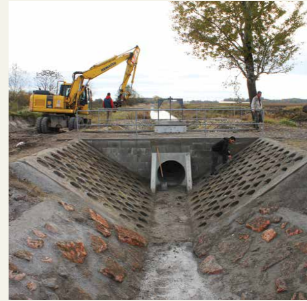
Sluice gates for water supply under construction | Photo: Tamás Gruber
