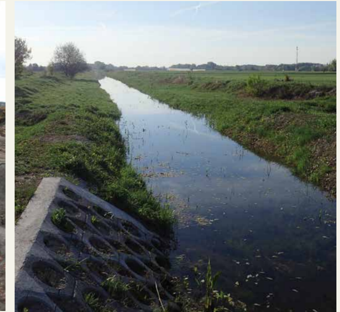
The water retention system in operation | Photo: György Verő
