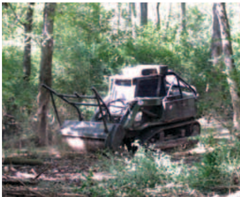
Fig. 1 – Privet was eliminated from 5-acre plots by hand-felling with saws (above) and machetes or by mulching with a Gyrotrac mulching machine (bottom). Residue was left where it fell.
