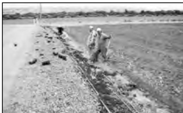
Installing short plants on a berm.
