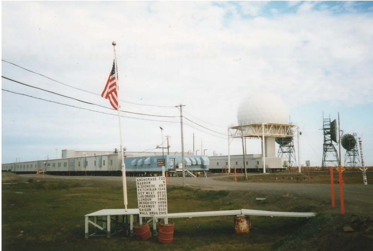
Figure 3.0 Ground Level View of Point Barrow LRRS
