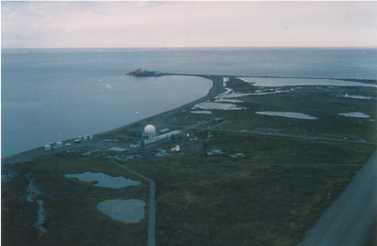
Figure 3.0 Aerial View of Oliktok LRRS
