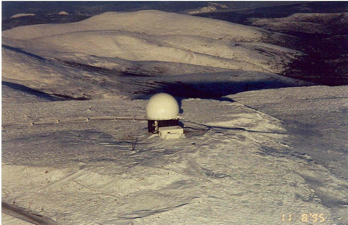
Figure 3.0 Aerial View of Indian Mountain LRRS Upper Camp
