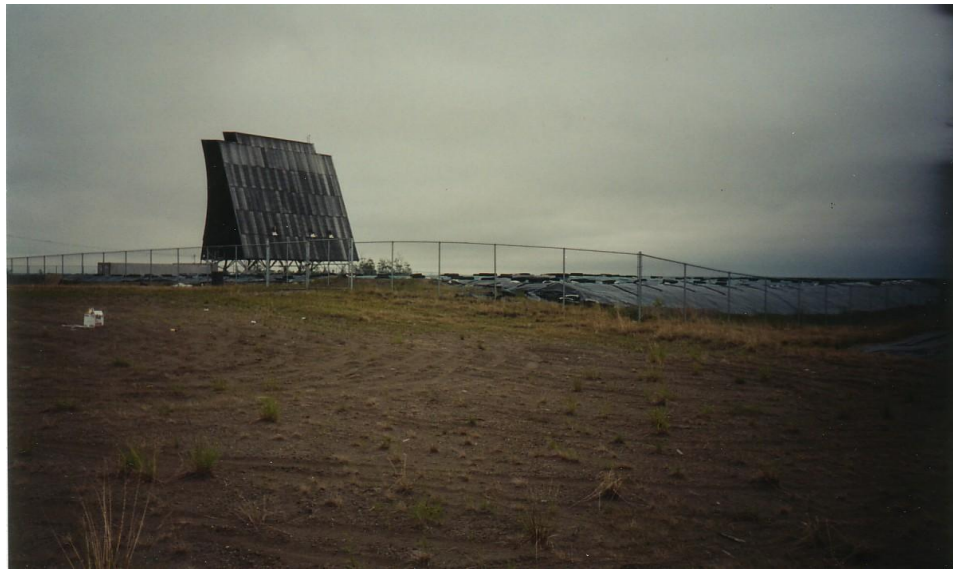
Figure 3.0 Ground Level View of Bethel Former RRS
