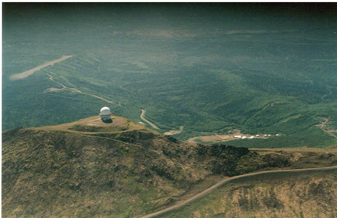
Figure 3.0A Aerial View of Tatalina LRRS
