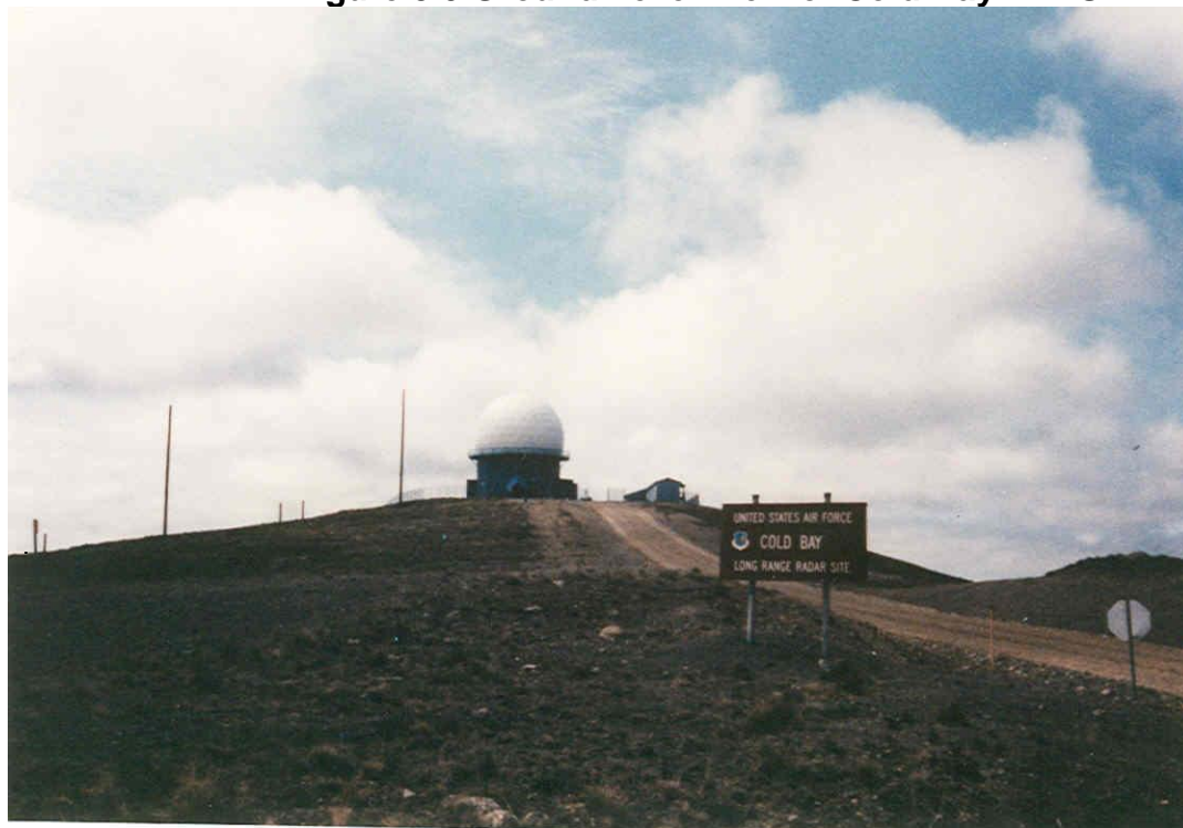
Figure 3.0 Ground Level View of Cold Bay LRRS
