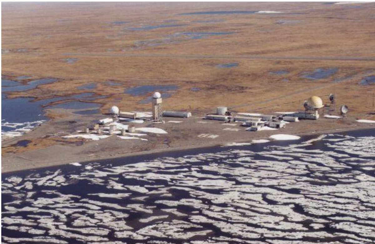
Figure 3.0 Aerial View of Bullen Point Former SRRS
