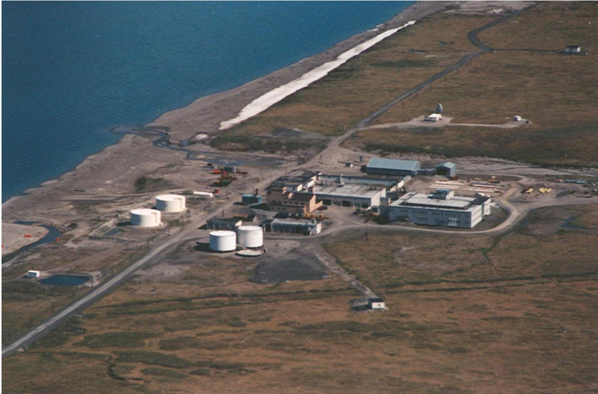
Figure 3.0 Aerial View of Cape Lisburne LRRS, Lower Camp
