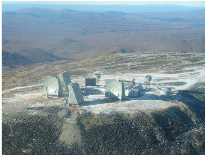
Figure 3.0 Aerial Views of Granite Mountain Former RRS, Upper Camp (Before and After Demolition)
