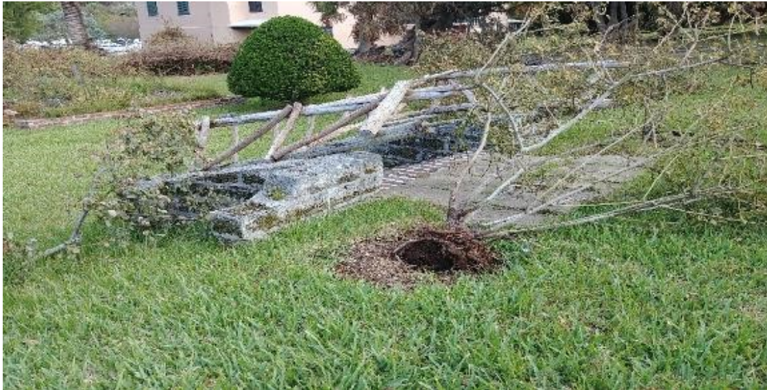
Damage to the south arbor at The Bermuda Rose Society Repository Garden at Waterville after Hurricane Humberto – September 2019
