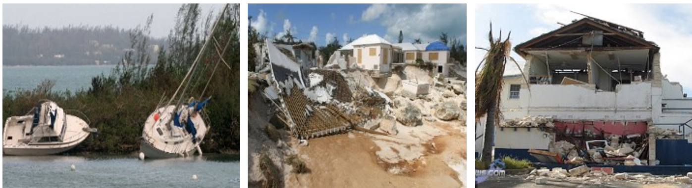
Damage after Hurricane Fabian - September 2003 (photos courtesy of Bernews.com)
