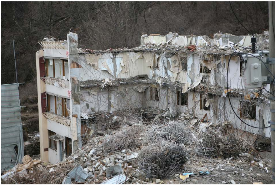
46 | Okin Apartments before and after demolition (© Okin Collective, 2012)
