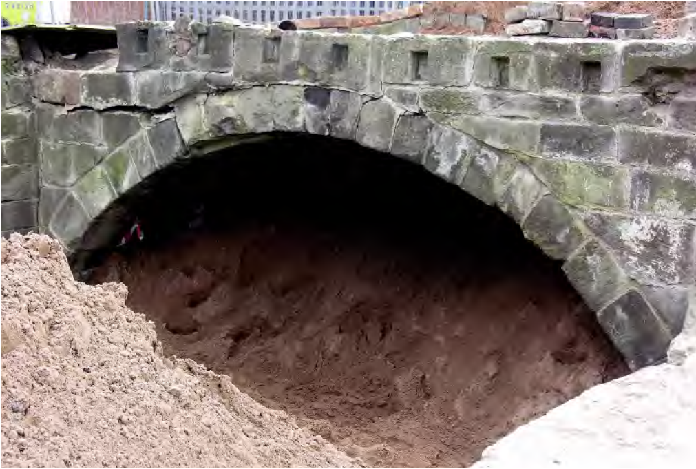
Fig 101 Partly infilled bridge arch, looking north-east
