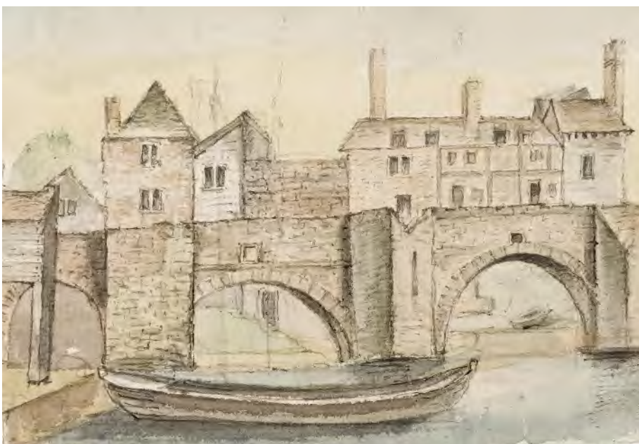
Fig 37 Watercolour of the northern end of the Welsh Bridge by an unknown artist, 1769, showing the west bastion, the open dry arch, the partly demolished gatehouse on the bridge and Frankwell Quay in the foreground, view looking east (SA, 6001/5326 fo 42; with permission of Shropshire Archives)
