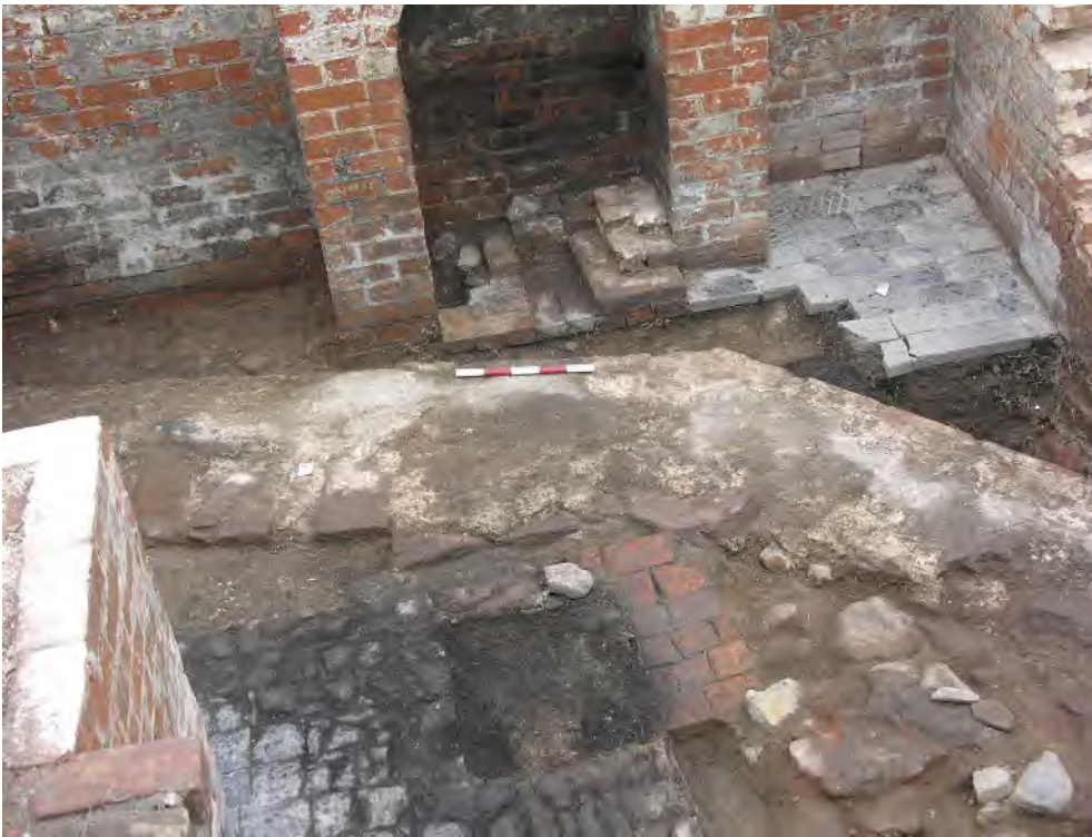
Fig 78 View of the stove position and area of intense contact on the north-west cellar (B18) floor, partly removed to expose the foreshortened east bastion (B8), looking east (0.5m scale)
