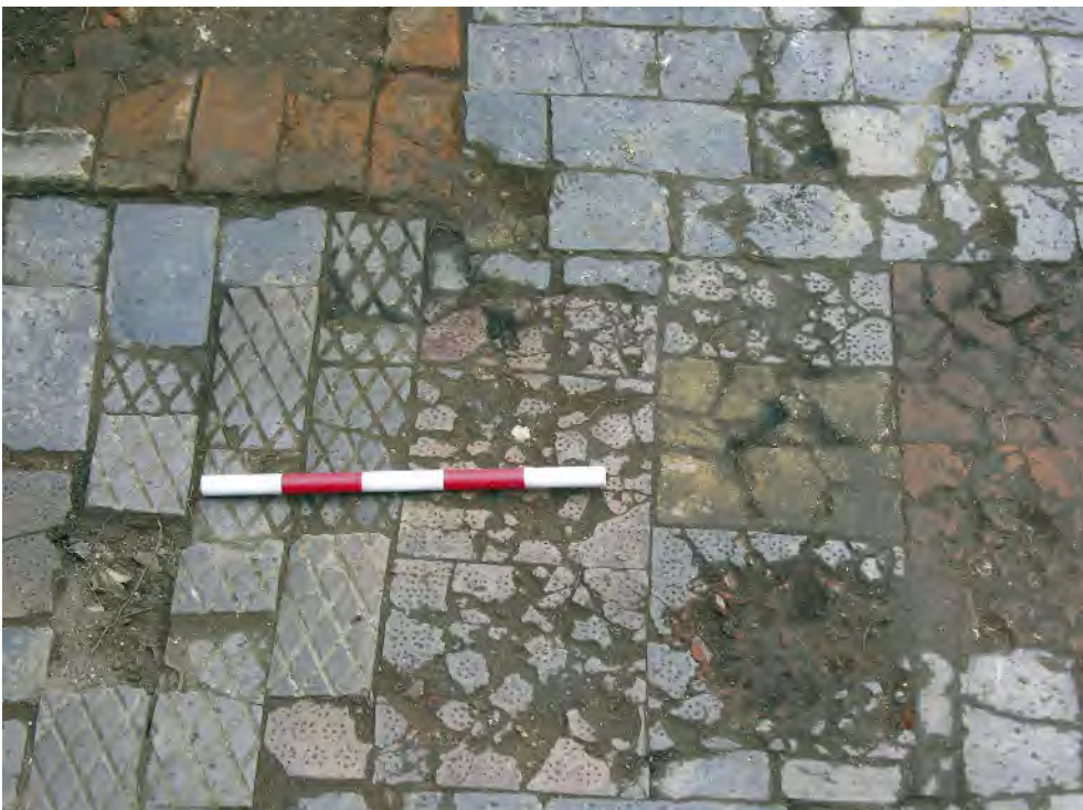
Fig 79 Rough repairs to the cellar floor of the south-west portion of Building 18, showing the degree of wear and the variety of ceramic tile and brick, looking west (0.5m scale)
