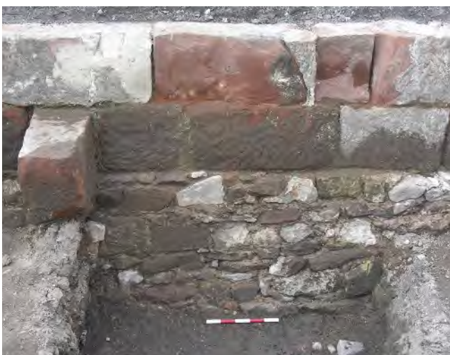
Fig 58 Detail of the ashlar and rubble foundation plinth of the barge quay and masonry abutment (S9), looking east (0.5m scale)
