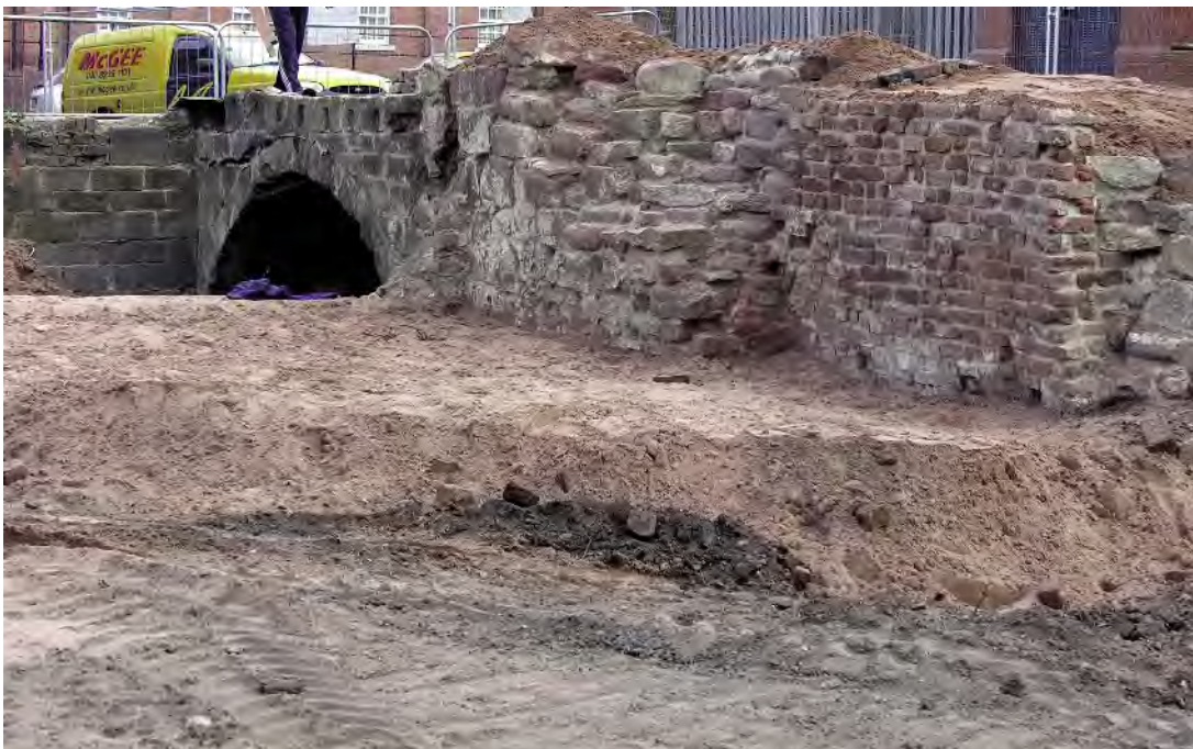
Fig 102 Reburial of the upstanding masonry in progress, looking north
