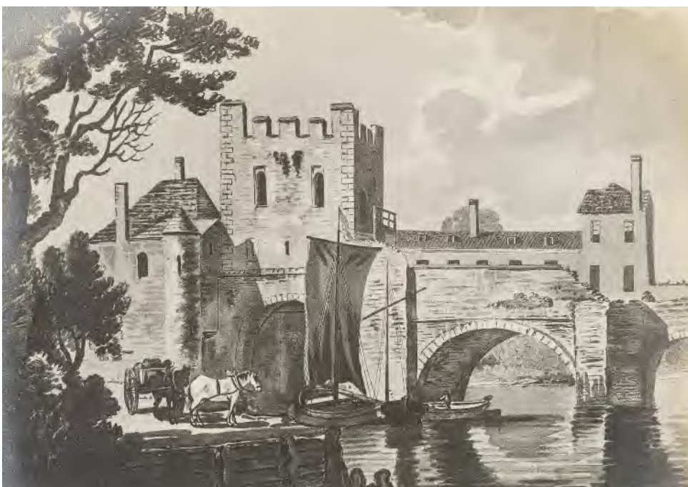
Fig 36 Watercolour based on a view of the northern end of the Welsh Bridge by Paul Sandby, c 1765–70, showing the dry arch and the gatehouse above, view looking east (SA, 6001/5326 fo 80; with permission of Shropshire Archives)
