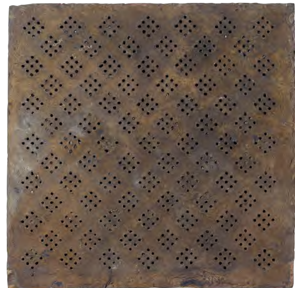
Fig 105 Malting kiln tiles reused as cellar floor paving, Building 18: with circular holes – <T14> (front and back views); with diamond holes – <T15> (front and back views) (scale c 1:3)
