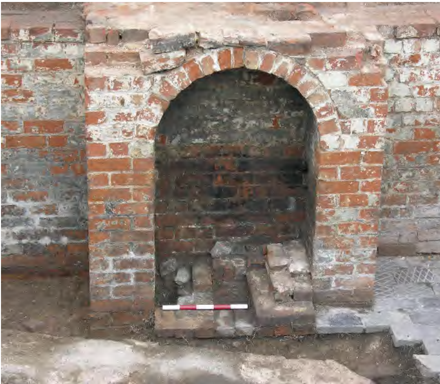
Fig 74 The fireplace in the north-west room of the cellar (B18), showing the later infilling partly removed, looking east (0.5m scale)
