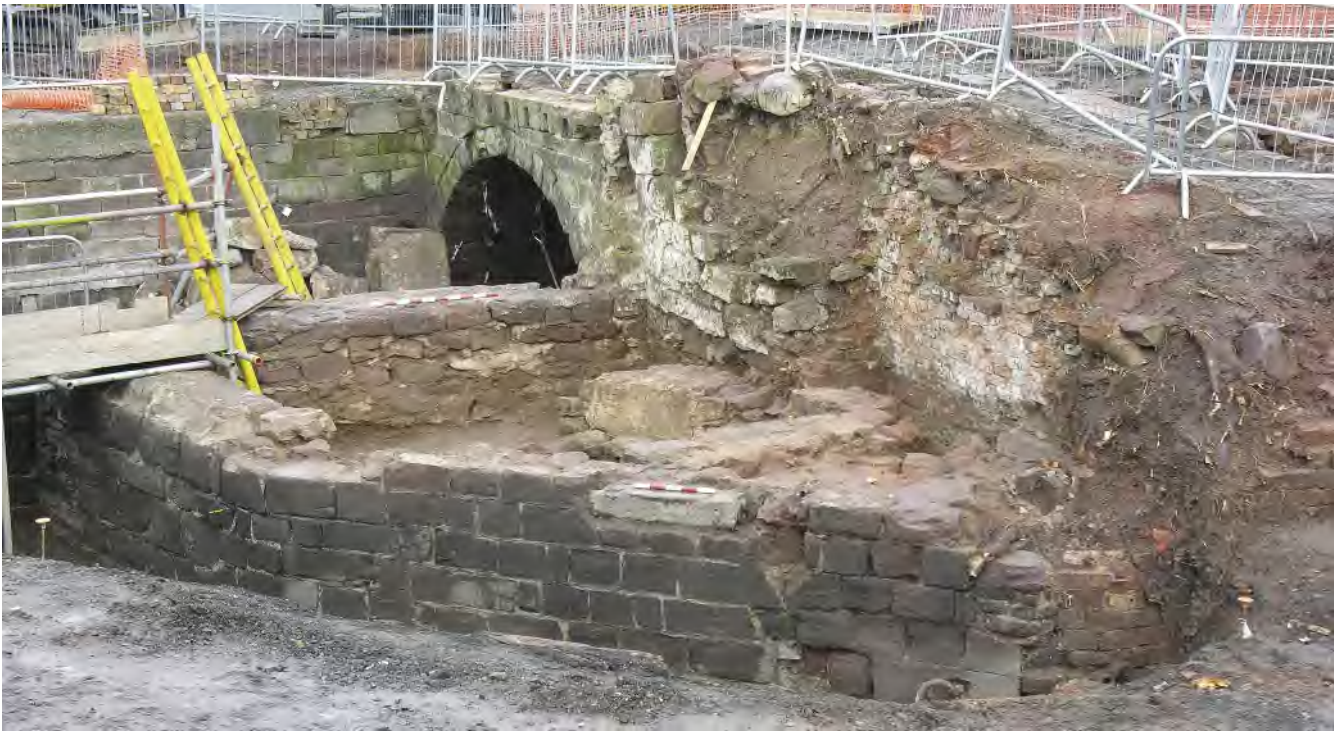
Fig 48 The external face of the western wall of the west bastion (B11), looking north (0.5m and 1.0m scales)
