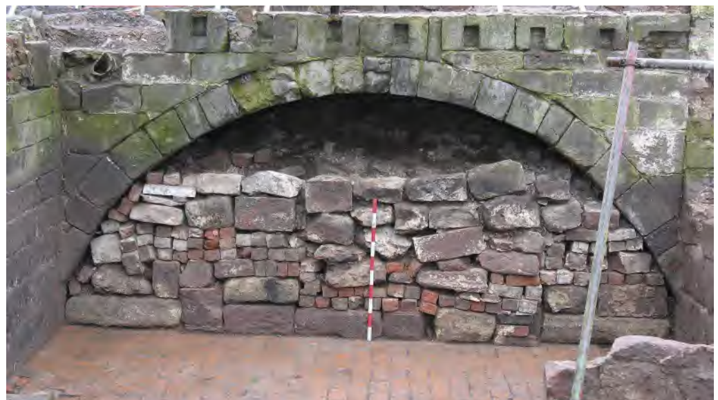
Fig 95 The ramshackle masonry wall, [22], which blocked the western side of the former dry arch (B9), looking west (1.0m scale)
