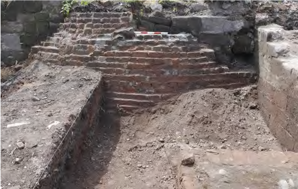
Fig 68 Brickwork blocking access to the eastern side of the dry arch (B9), looking west (0.5m scale)
