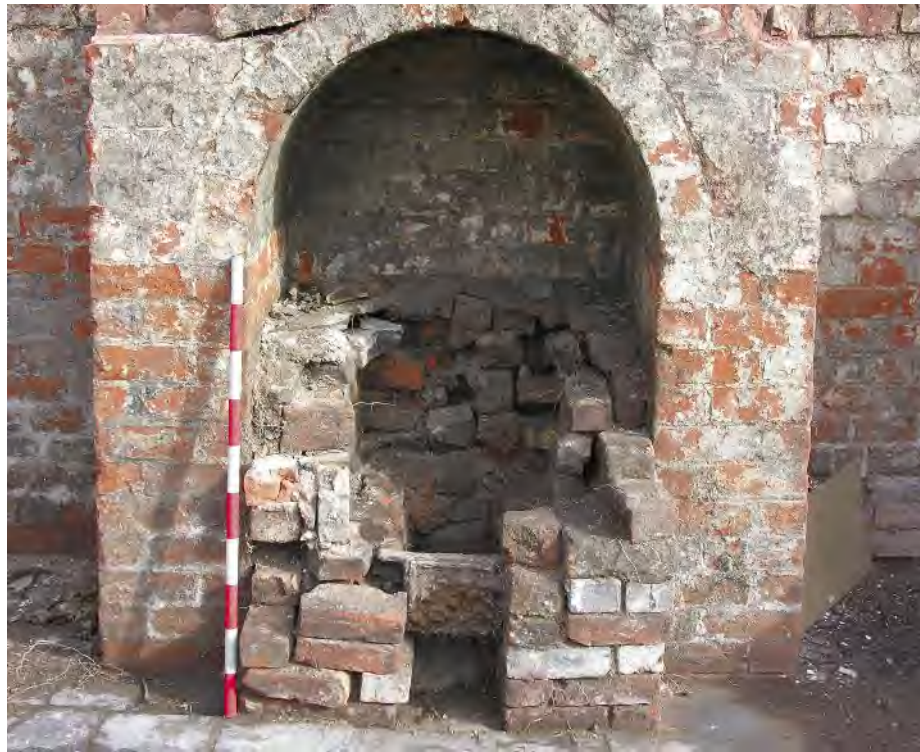
Fig 76 The basal portion of the grate or stove later inserted in the fireplace in the north-west room of the cellar (B18) (1.0m scale)
