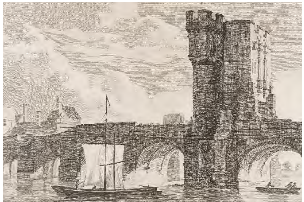
Fig 42 Print of the central portion of the Welsh Bridge in 1776, showing the two phases of the Mardol Gate and the buildings on the eastern side of the bridge, view looking east (SA, 1220/3; with permission of Shropshire Archives)
