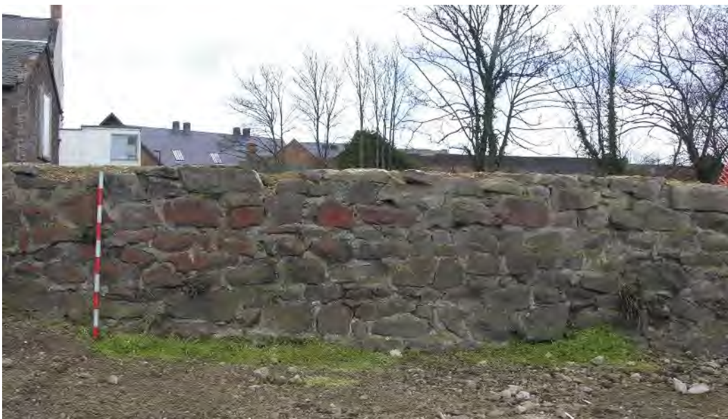
Fig 82 Central portion of the western boundary wall [48], looking east (1.0m scale)
