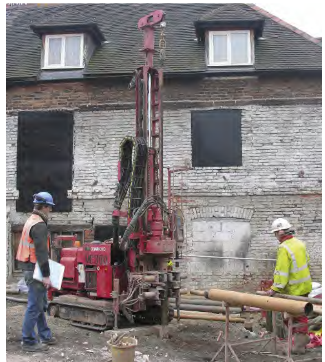
Fig 8 Undertaking the geoarchaeological survey with the MC300 drilling rig
