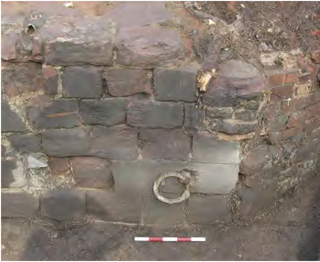
Fig 50 The south-west corner of the west bastion (B11) showing the location of mooring ring [163], looking east (0.5m scale)
