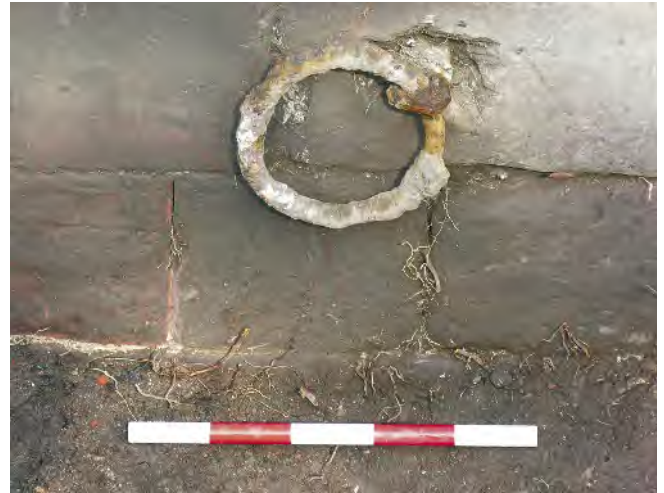
Fig 51 Detail of mooring ring [163] on the south-west corner of the west bastion (B11), looking east (0.5m scale)
