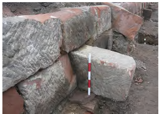
Fig 59 Detail of the protruding ashlar block in the external (eastern) face of the barge quay and masonry abutment (S9), looking north (0.5m scale)
