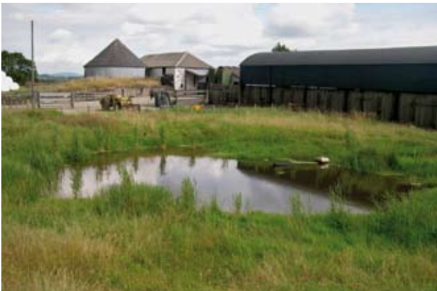
A recently created sustainable farm drainage pond at Barnboard Farm, Bridge of Dee, August 2006. (Peter Norman)
