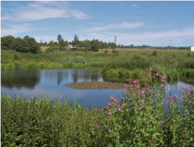
Brieryhill sustainable urban drainage scheme. Lockerbie, July 2006. (Peter Norman)
