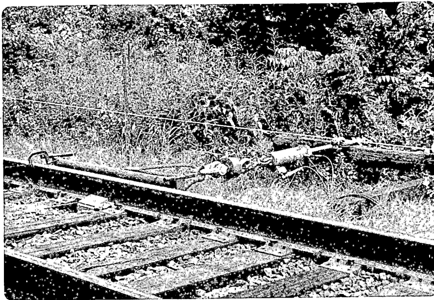
Fig. 18 - PULLING THE TRACK PANEL
