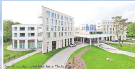
Swinemünde, Hotel Interferie Medical Spa
