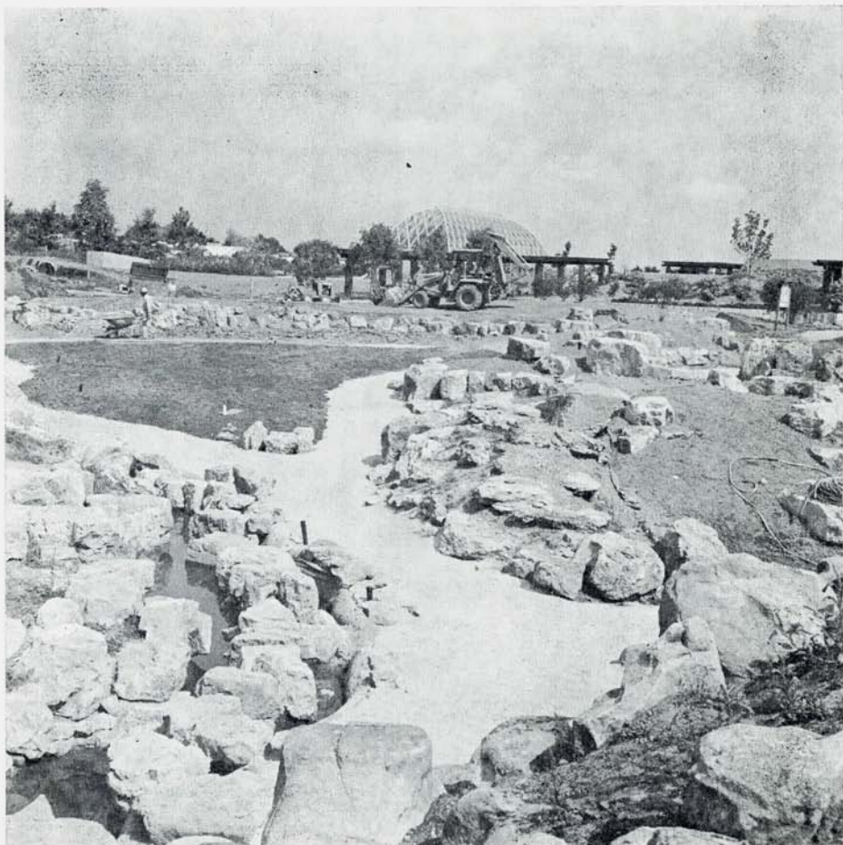
Nearing end of construction — October, 1979
