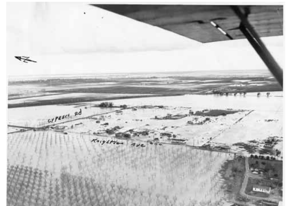
Figure 3.15. Marsh Creek flooding. (below) This picture shows flooding in the very northeast corner of ECCC, at the edge of the historical tidal marsh and looking east across the Delta. This area would have been part of the natural overflow zone of Marsh Creek. (Image courtesy of Contra Costa County)
