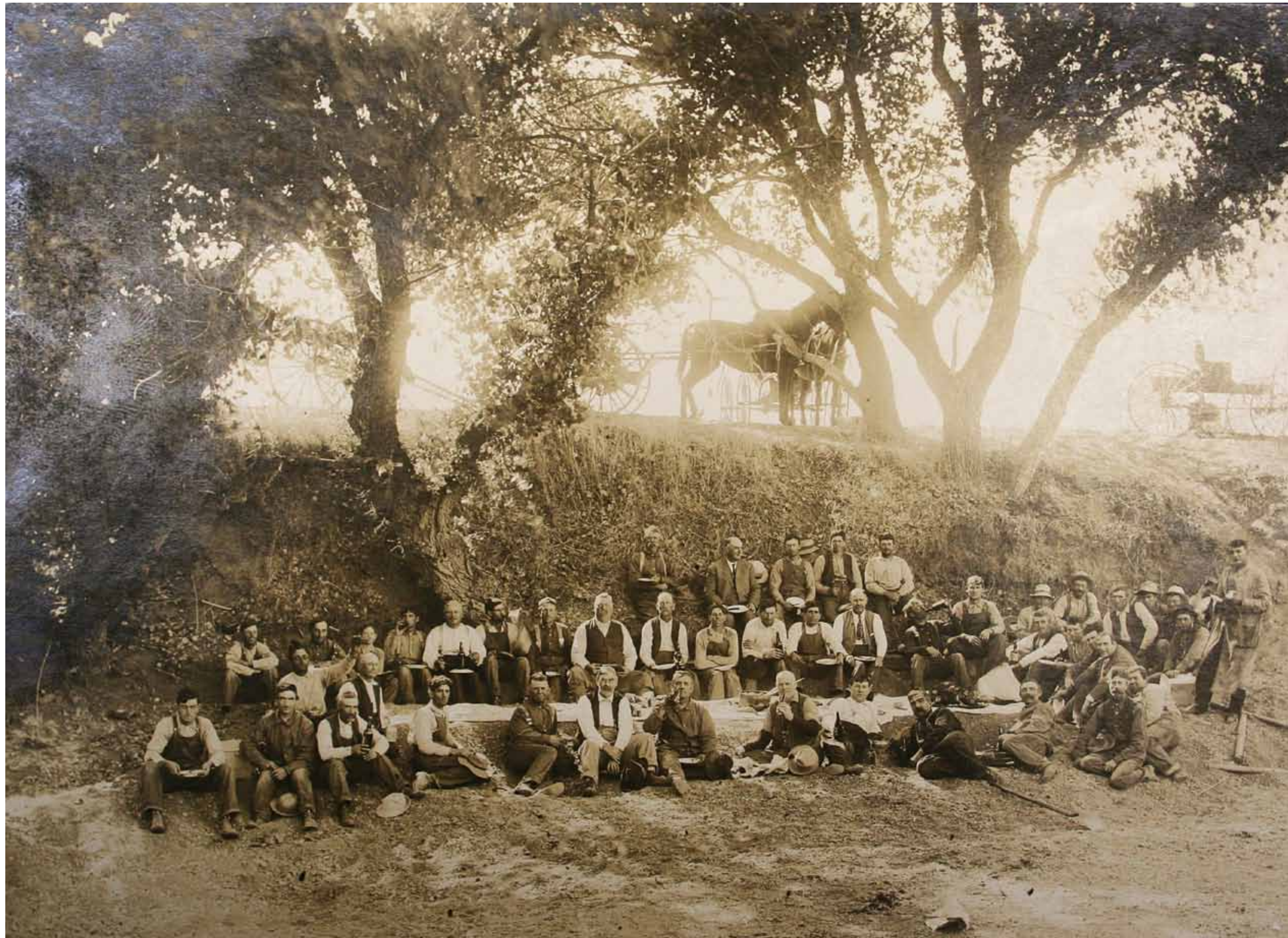
Figure 3.8. Gravel mining in Marsh Creek. This early photograph is titled “Gravel for Lone Tree Way. Taking it out of Marsh Creek.” The removal of gravel from the creek likely contributed to incision and bank erosion. (Unknown ca. 1905, courtesy of the East Contra Costa Historical Society)
