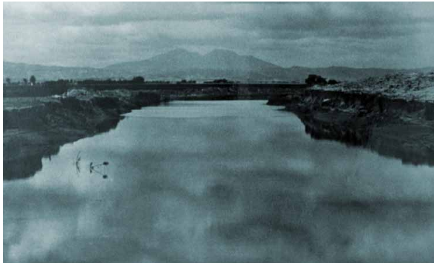
Figure 3.9. Two canals. Canals such as these were dredged to carry water to and from the San Joaquin River. At left, “Dredged canal connecting with Indian Creek” (likely a reference to Indian Slough) shows a canal that provided irrigation water. At bottom, “View of Kellogg Creek ditch of the Byron-Bethany irrigation district,” shows Kellogg Creek channelized to carry flood water rapidly away from farmland to the San Joaquin River. (Left: Unknown n.d., courtesy of the Antioch Historical Society; Bottom: Unknown n.d., courtesy of the Pittsburg Historical Society)
