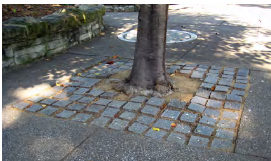
Tree grates (top and middle) and pavers (bottom) are often used for street tree plantings
