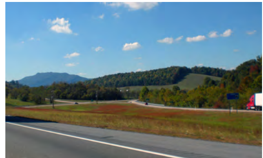
Use grasses or other low-growing vegetation to preserve views, like this interchange at exit 50 on Interstate 81 in Washington County
