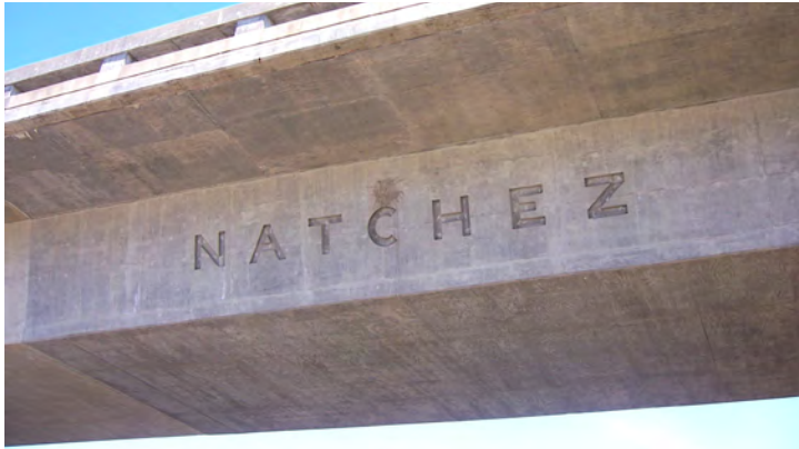
Natchez Trace Parkway bridge with engraved concrete
