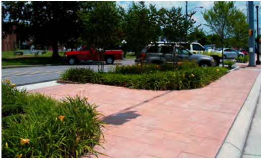
Colored and stamped concrete sidewalk
