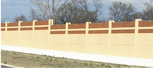
Color treatment on a noise barrier
