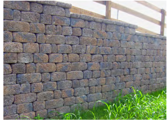
Modular block can be made to resemble real stone by using various textures and color additives
