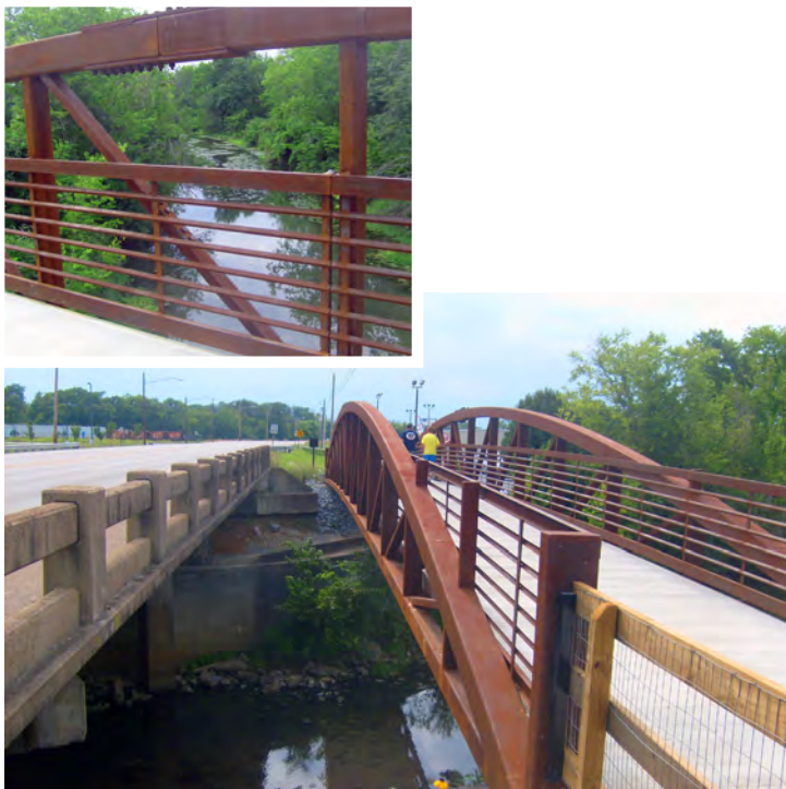
Weathering steel, like this pedestrian bridge in Lebanon, Tennessee, complements the natural environment
