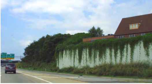
The vines cascading down this retaining wall and the vegetation at the base soften the wall's appearance
