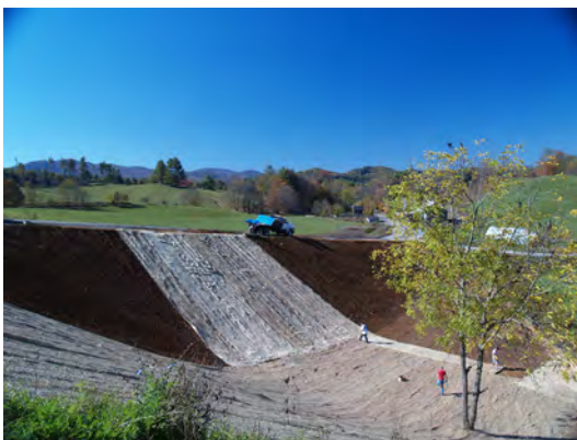
Installation of an erosion control blanket
