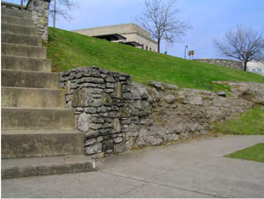
Manmade walls are integrated into exposed limestone using stone with similar characteristics
