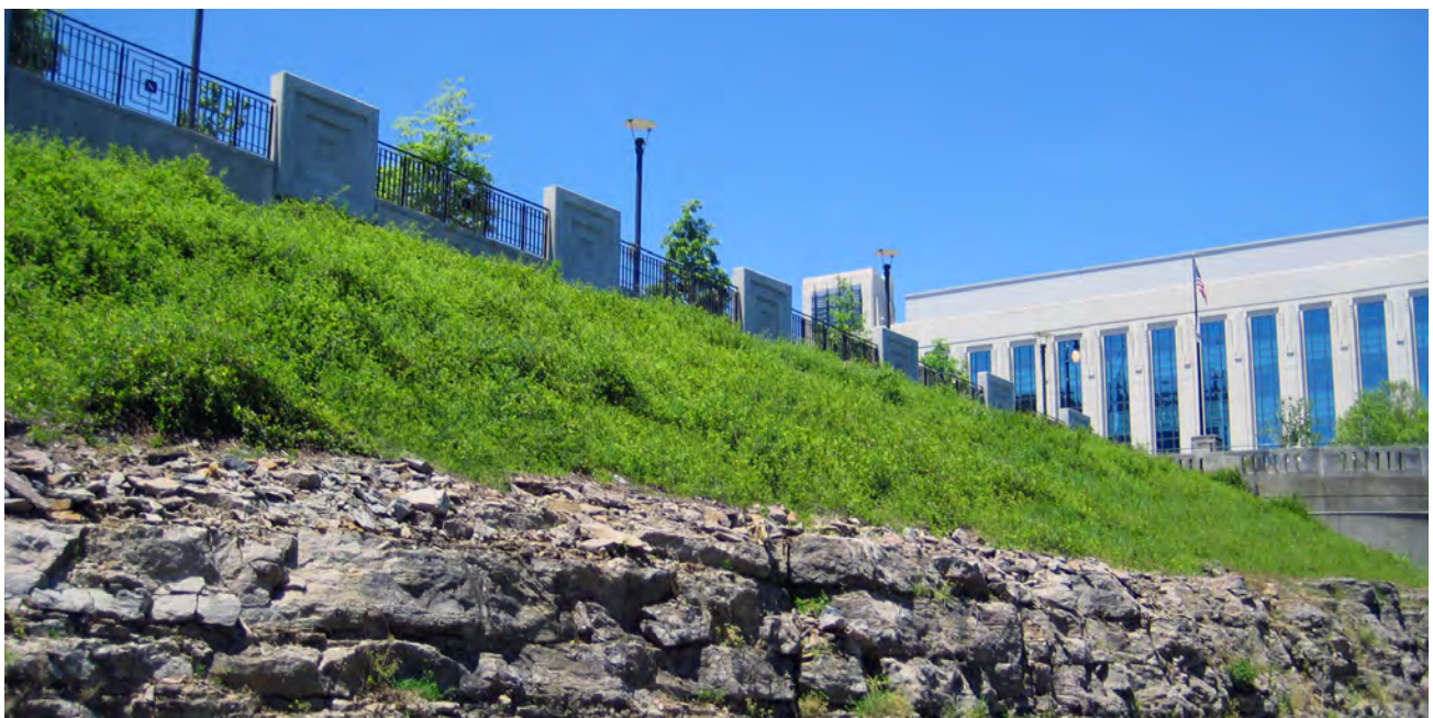
Spreading shrubs, like these Cherokee roses, are an excellent ground cover for slopes and areas that are inaccessible to maintenance equipment
