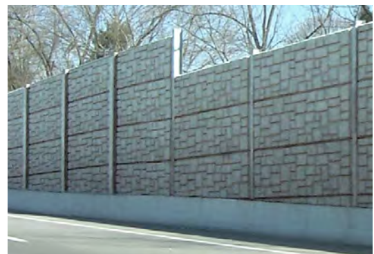
Stamped concrete can be used on horizontal surfaces (top), vertical surfaces (bottom)
